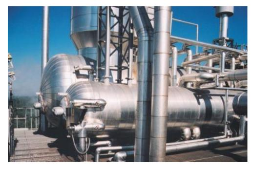
Chemical enterprises are using vapor for cleaning, drying, fermentation, stripping and so on. Local vapor (SIP) is a widely used method for sterilization in pipes, including on-line sterilization of containers, valves, production lines and filter assemblies, etc. Vapor is produced within the boiler, where hot water is converted into vapor under pressure.
