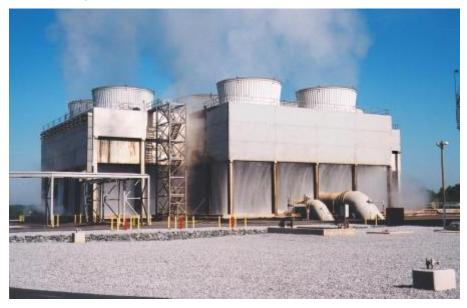
Open system cooling towers remove waste heat from the vapor cycle by exposing the cooling water directly to the atmosphere. After evaporation removes the heat, the remaining cooling water flows into thce catch pool. Level control applications include a high level switch to avoid overflow from the cooling tower pool. In DC cooling systems, the inlet structure is usually a vertical sewage well pump, which requires high and low water level detection and possible pump control.
