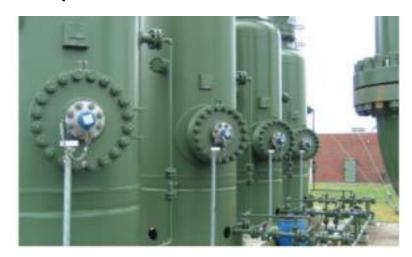
Natural gas can traverse thousands of kilometers of pipelines. Compressors placed in critical intervals can maintain natural gas even and reliable transmission. A typical compressor station includes an inlet scrubber to collect liquids and residues that may form in the gas pipeline. The washing tower includes a main device and a secondary device. The liquid and solid parts are separated from the air flow in the main device, and the secondary device is responsible for removing oil mist.
